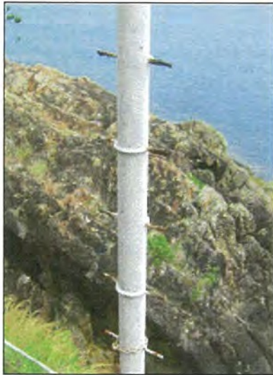
Photograph 23: Replace existing climbing rungs to central winch arm
