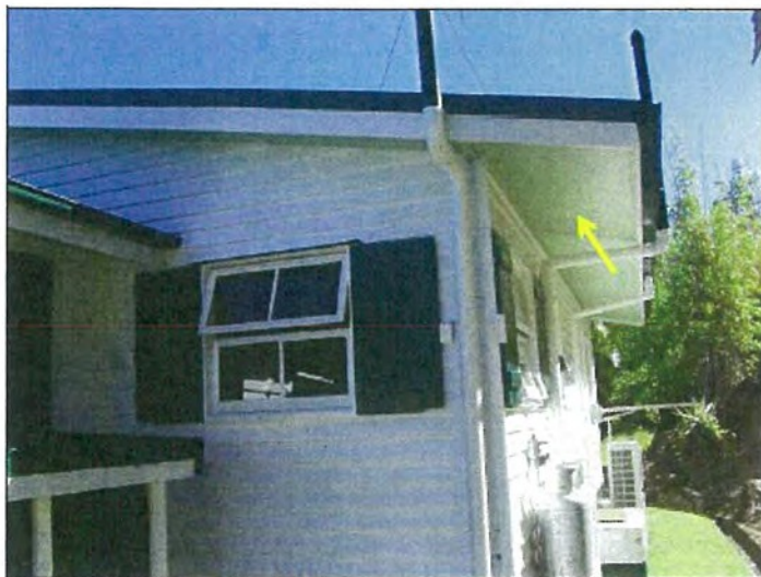
Photo S-7500: Eave soffits cladding
