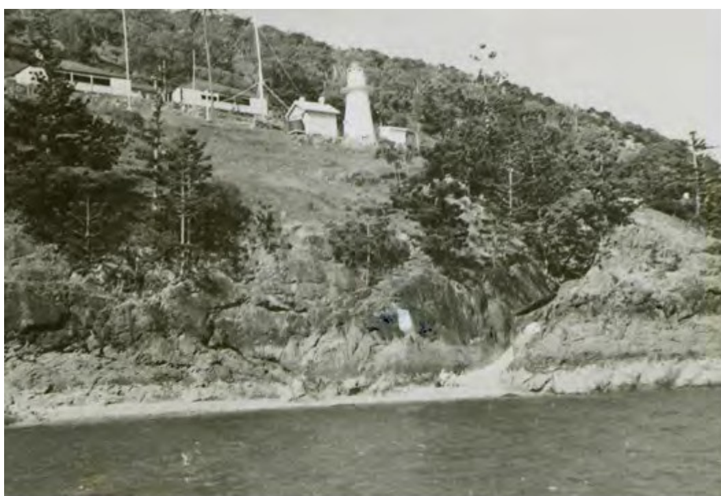
Figure 8 — The lightstation, c. 1950
