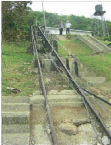
Photograph 15: Winch trolley rails and supports
