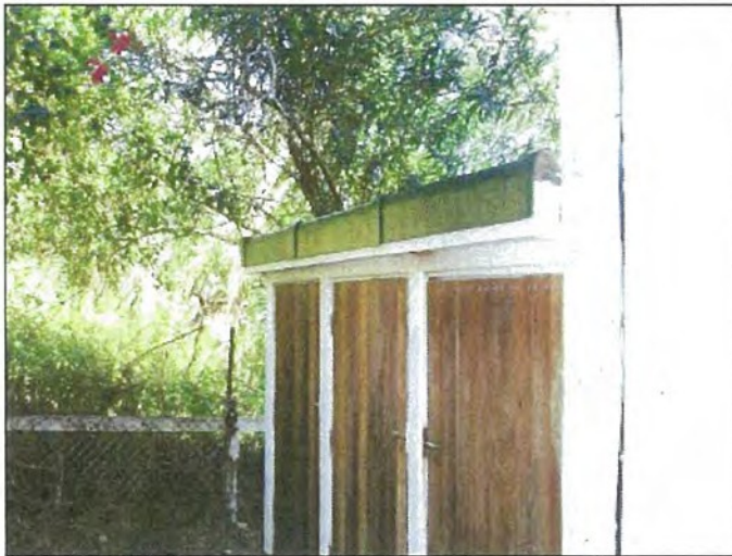
Photo S-7518: House 2: storage shed, edge capping on roof peak
