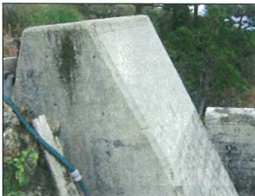
Photograph 10: Concrete derrick crane anchor block
