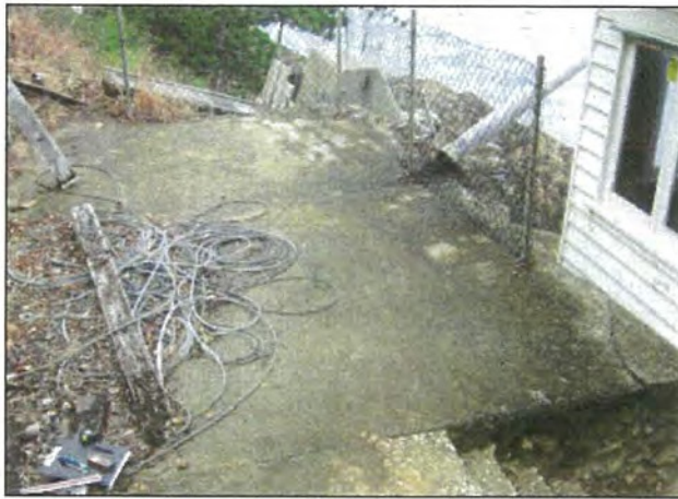
Photograph 5: Concrete platform to front of winch house
