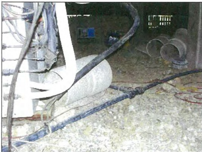
Photo S-7505A: Stored vent pipe pieces under House 1, Northern end
