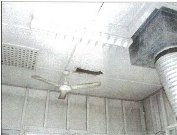
Photo S-7511B: Internal ceiling cladding in Gen. Shed
