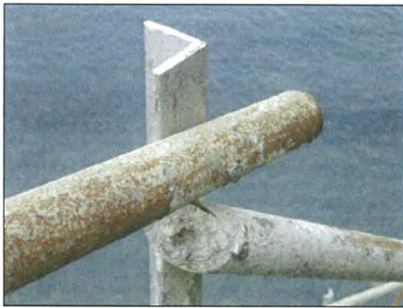
Photograph 26: Isolate dissimilar metals
