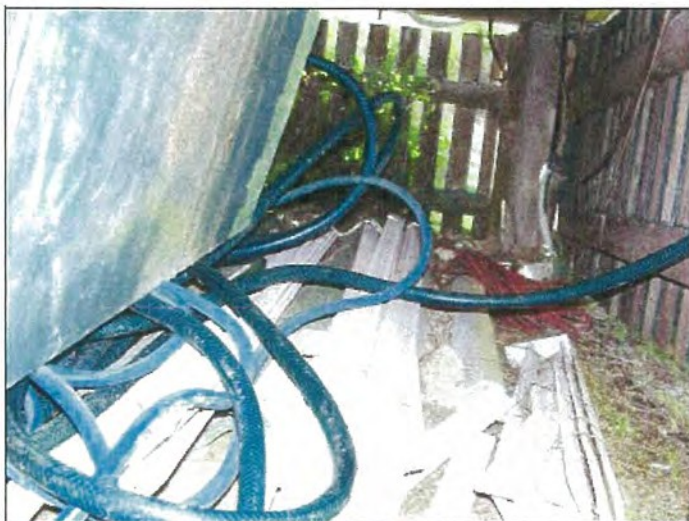
Photo S-7508: Flat & corner cover strip mouldings under House 1, Southern end
