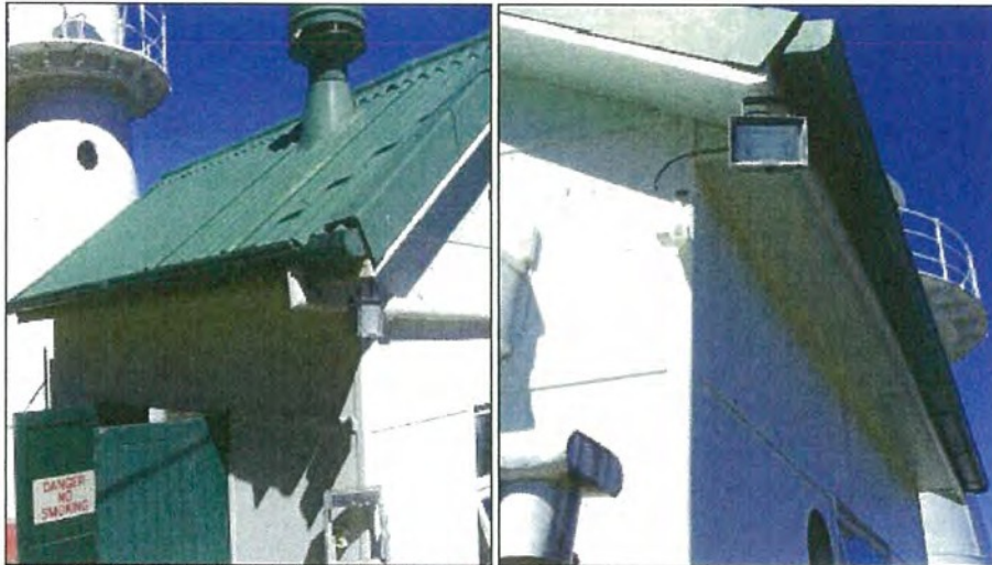
Photo S-7513: Guttering on East & West sides of Gen. Shed
