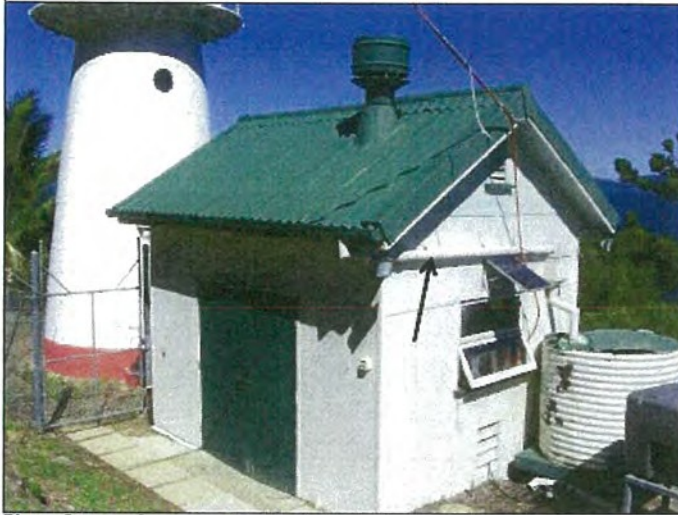
Photo S-7512: Generator Shed, rainwater pipe Photo S-7497D: Roofing sheets; Photo S-7498E: Edge capping; Photo S-7507D: Ridge capping Photo S-7505B: Air vent on roof; Photo S-7511B: External wall cladding; Photo: External flat & corner cover strips
