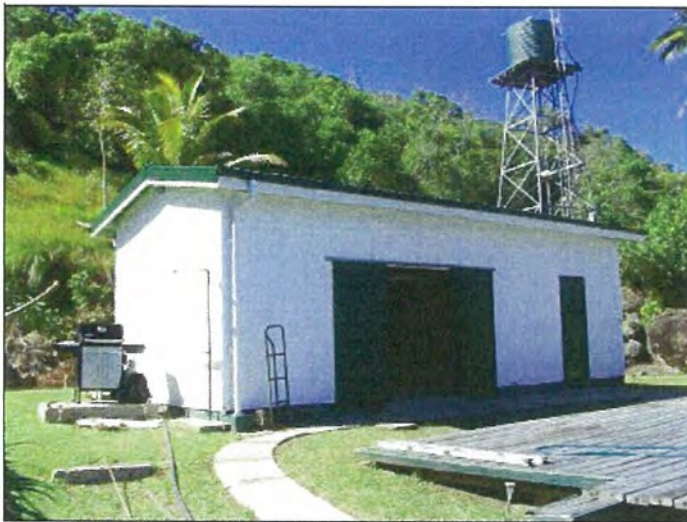
Photo S-7509: Workshop Shed, flat cover strips Photo S-7510: corner cover strips Photo S-7511: wall cladding
