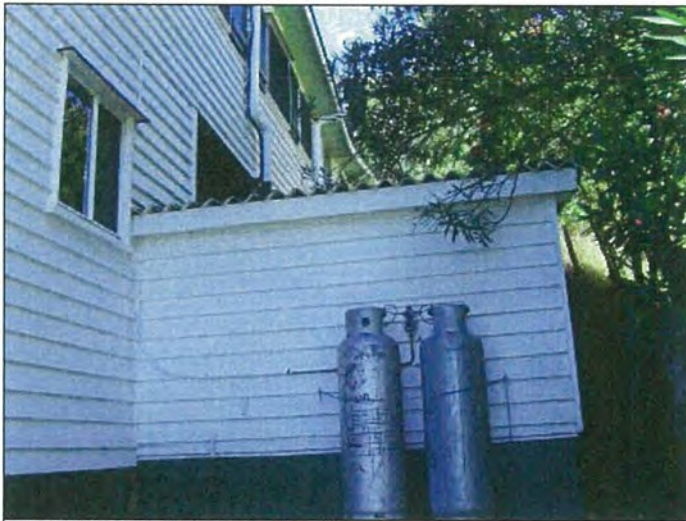
Photo S-7520: Roof sheets on storage shed
