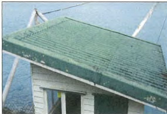
Photograph 4: Existing roof cladding
