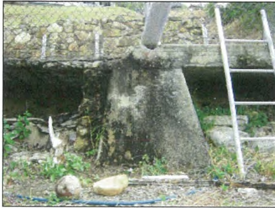
Photograph 25: Fill cavity under suspended landing slab
