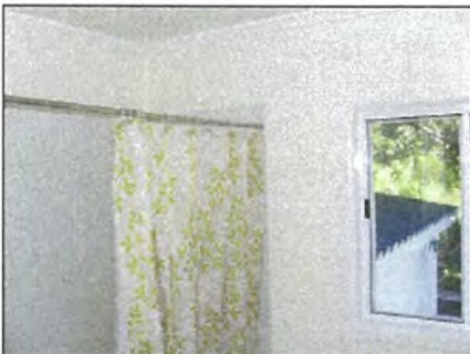
Photo S-7525: House 2, Bathroom, walls in bath / shower section only
