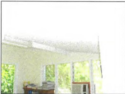
Photo S-7523: House 2, half ceiling in Office
