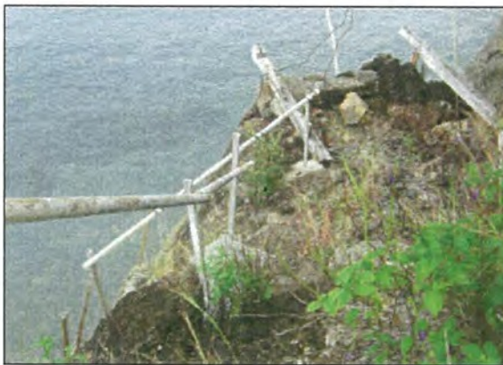
Photograph 14: Access handrail down to water
