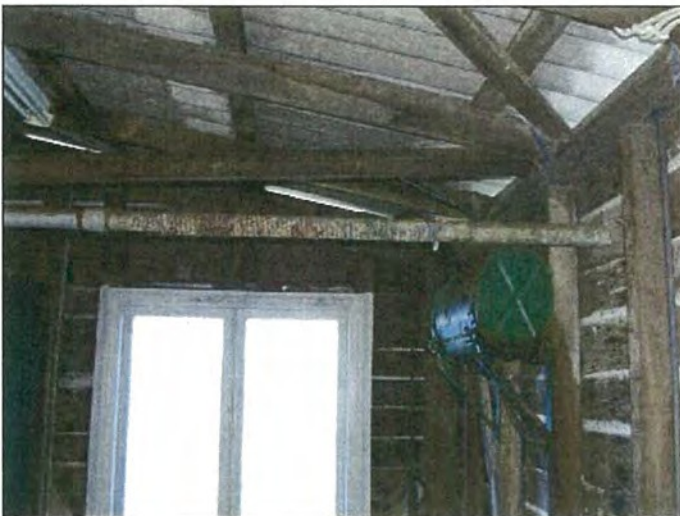
Photo S-7515: Winch House, remnant lagging on pipe
