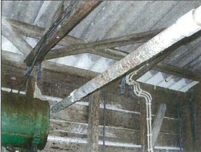
Photo S-7515: Winch House, remnant lagging on pipe
