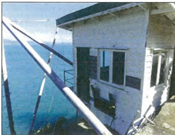
Photograph 2: Dent Island Winch House
