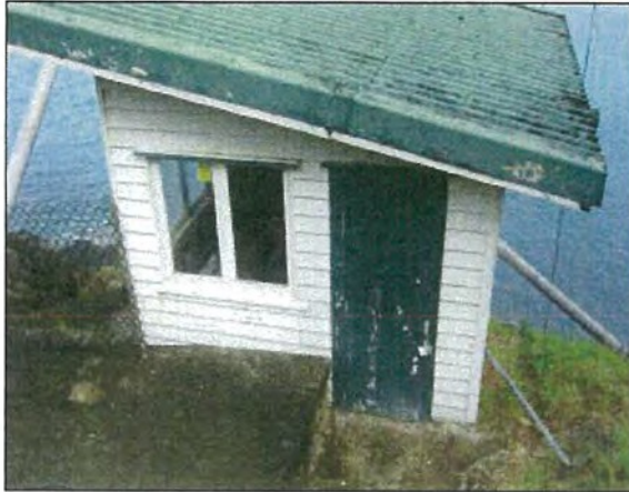
Photograph 16: Winch house to be painted
