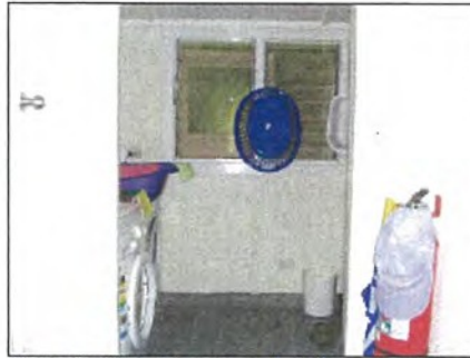
Photo S-7524: House 2, wall cladding beside Laundry tubs, one wall only
