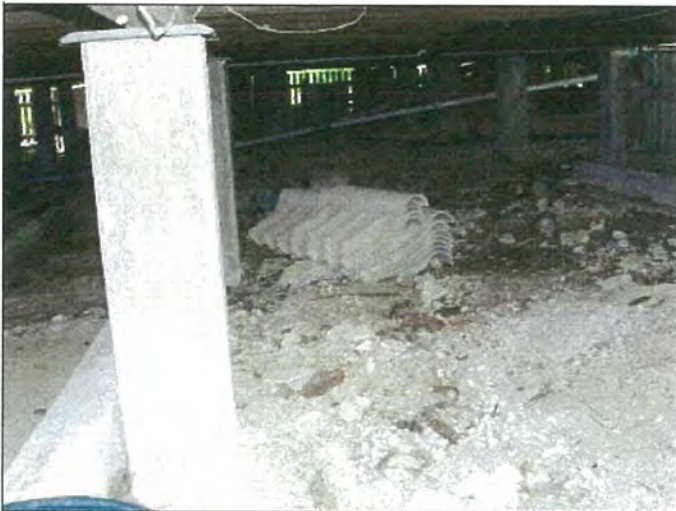
Photo S-7507A: Stored ridge capping under House 1, South East end
