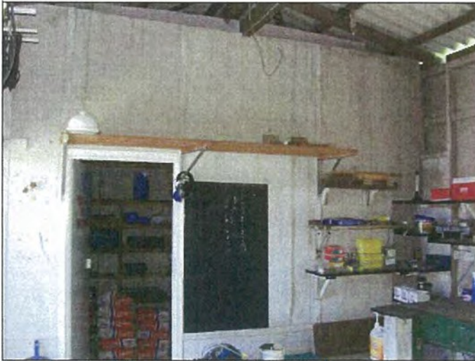
Photo: Internal wall & flat cover strips, Workshop Shed
