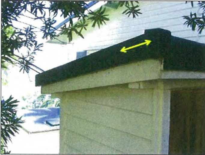
Photo S-7519: Edge & corner capping on roof of storage shed
